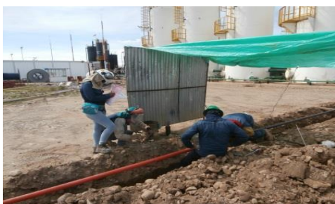
Fot 9. Supervisor HSE
