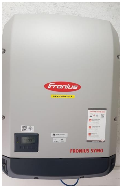
Inversor Fronius On-Grid de 15 kW
